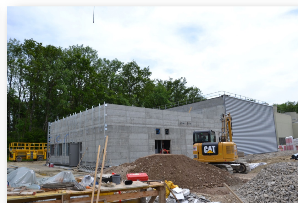
Figure 2. Worksite status in June 2014.
