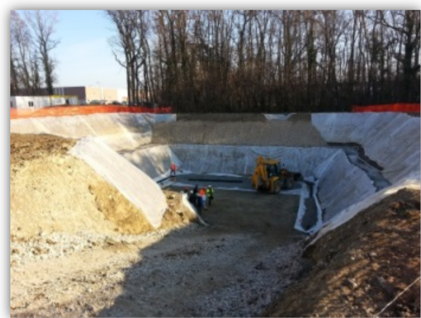
Figure 1. Worksite status in November 2013.
